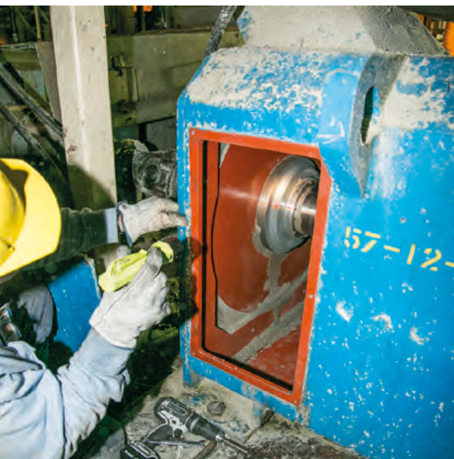
Inspecting the recently installed AEGIS® PRO Series Bearing Protection Ring on a key motor at the Midwest paper mill. Designed to close around the motor shaft, the split-ring PRO SL was installed without decoupling the motor.
